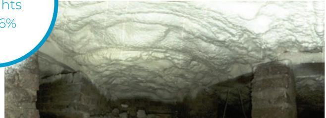
Fig 9. After the installation, showing the insulation now applied.
